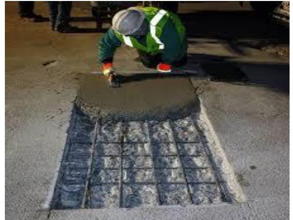
Fig 5.1.4.3 Repairing corrosion damage material
