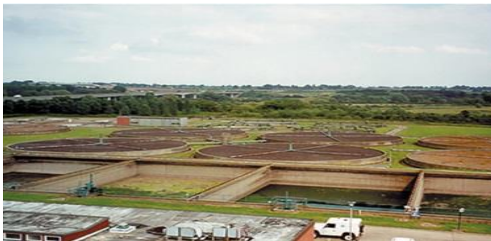
Fig 5.1.9.2 Filter beds at a waste water treatment plant
