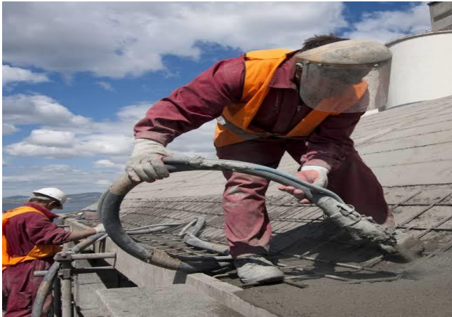
Fig 5.1.4.3 Repairing corrosion damage material
