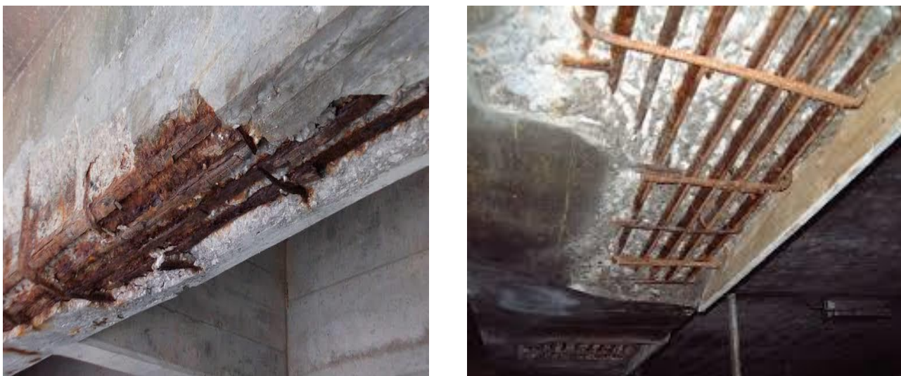
Fig 5.1.4.1 Effect of corrosion in reinforcement
